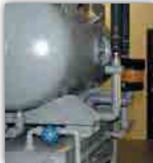
Watchdog Breather installed on a hydraulic reservoir
