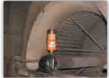
Grease lubricator installed on a blower fan
